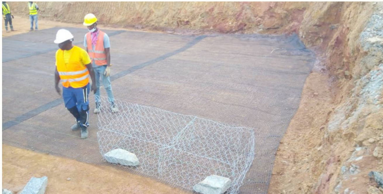
2. Placing gabions and laying geogrids
