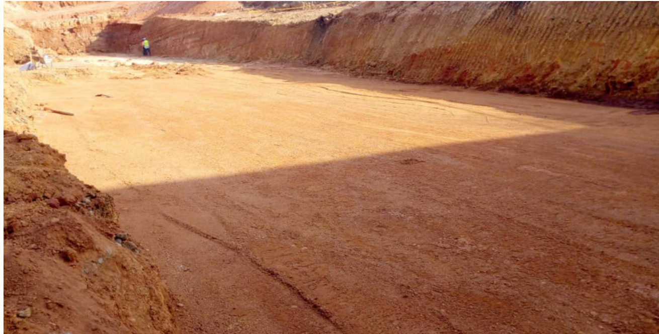
1. Excavation and ground preparation
