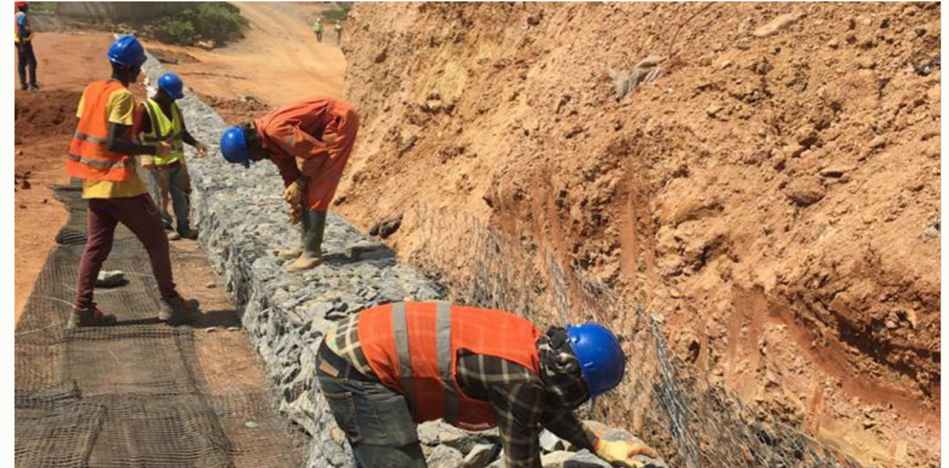
3. Filling the gabions with rocks
