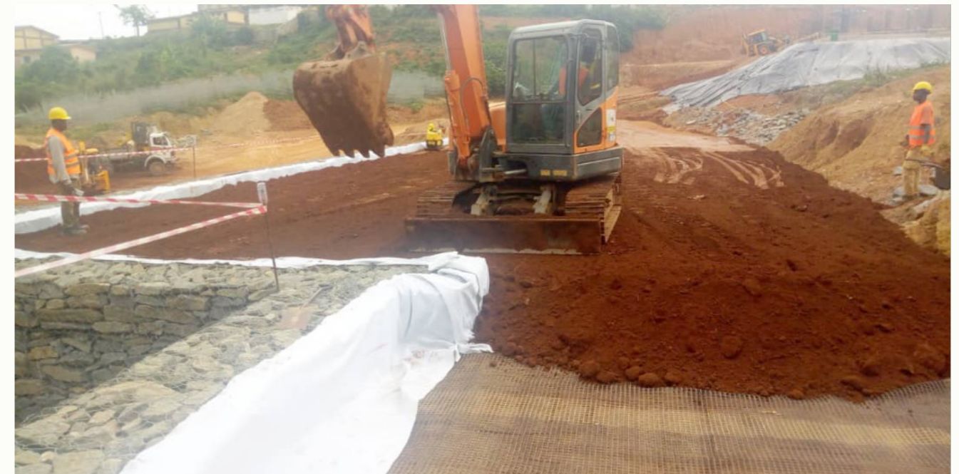
4. First layer of 25 cm thick backfill material
