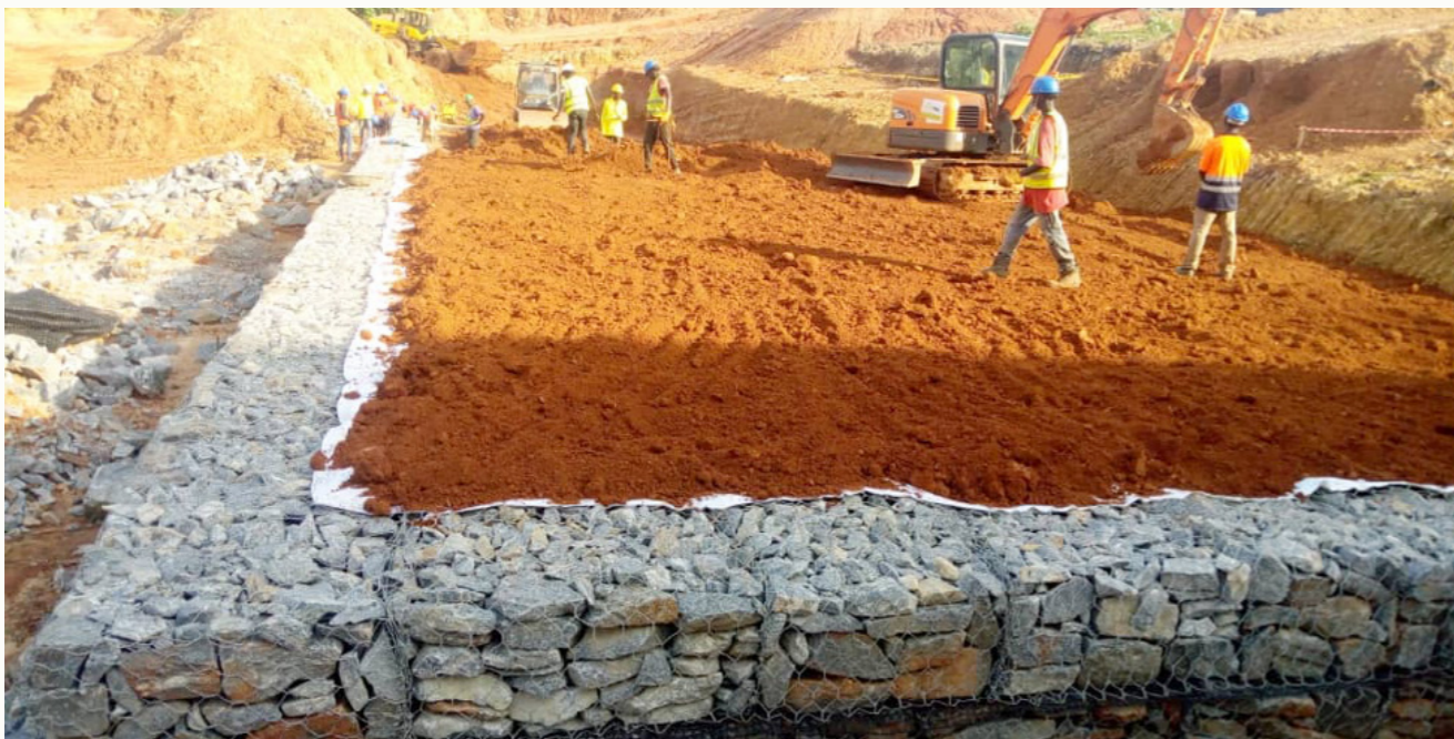
6. Second layer of 25 cm thick backfill material
